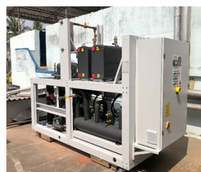
Compressor rack installed at an identified seafood industry, Cochin
